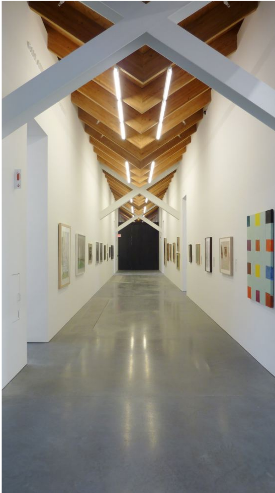
Steel braces punctuate the "spine gallery". Photo: Christopher French
